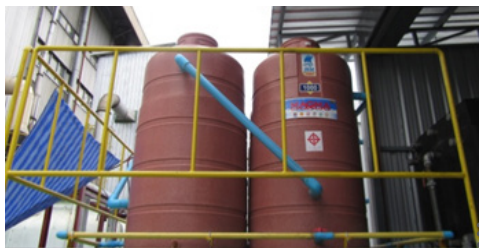
Enhance wastewater treatment system
